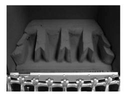
b) Position the two halves of the front ceramic (L/H & R/H) on the locating channel in the front ceramic, ensuring it is located onto the lip on the burner front ceramic support. (See fig. 2 below)
